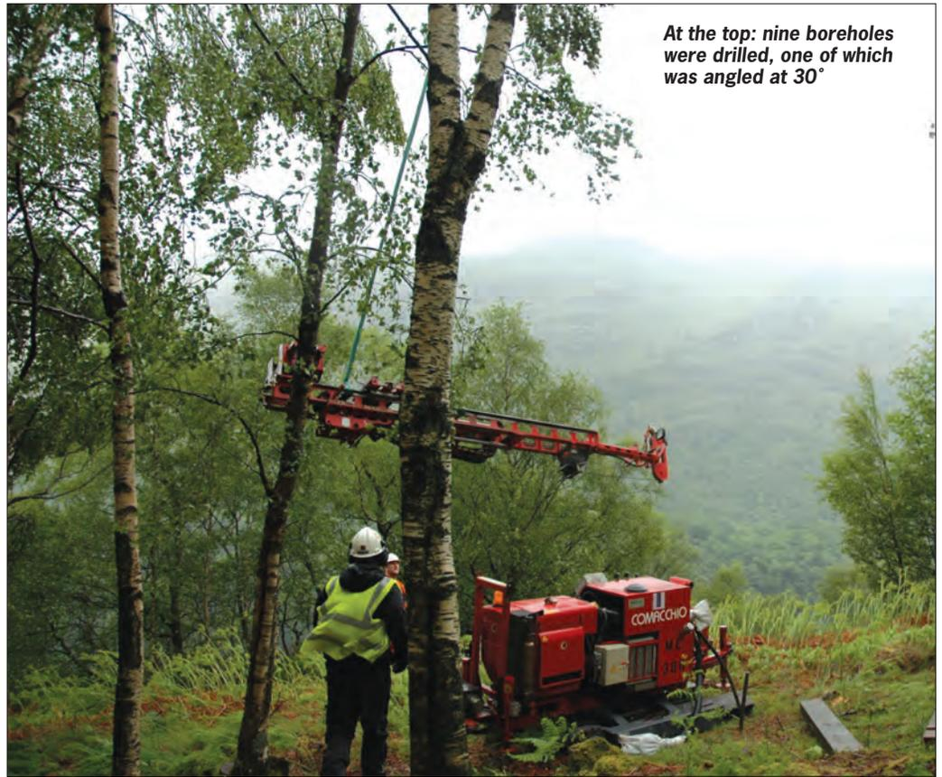
At the top: nine boreholes were drilled, one of which was angled at 30°
