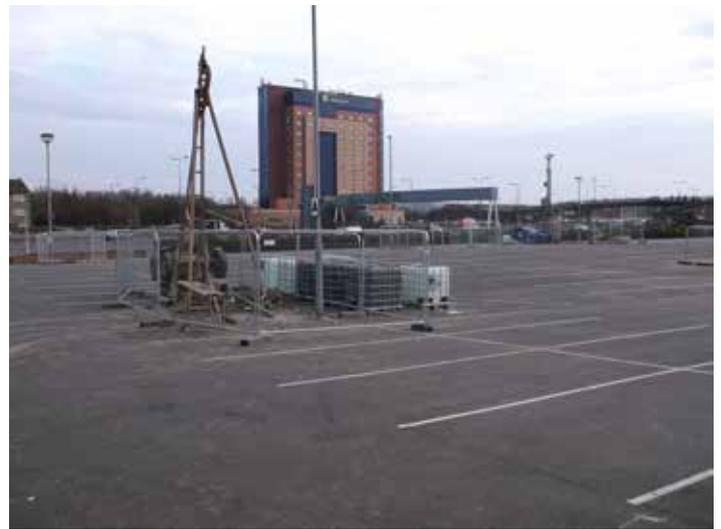
Boreholes were drilled into the London Clay using cable percussion rigs
